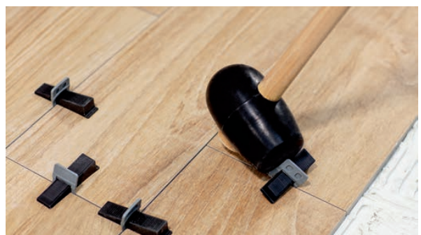
6 Retirar sistema / Retier le systeme / Remove the system
