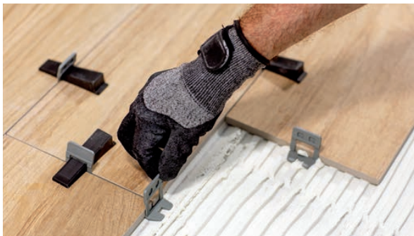
1 Colocar bases / Placer les bases / Place the base
